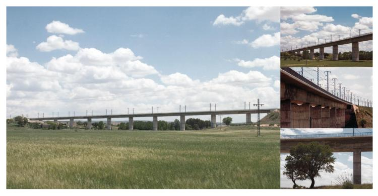
This structure consists of 11 spans of 30.00m + 9 x 45.00m + 30.00m. The bridge is 13.00m wide therefore permitting a two-way high-speed railway line.
